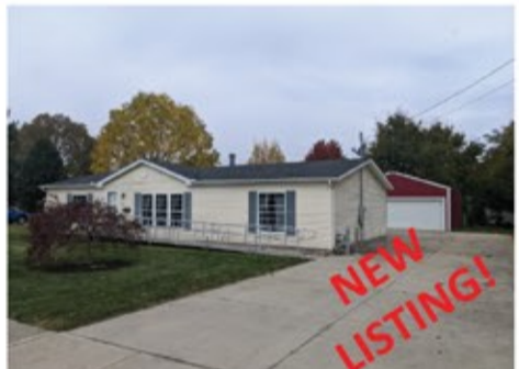
NEW LISTING! 3 Bed 2 Bath, Pole Barn w/concrete floor Cardington $164,700
